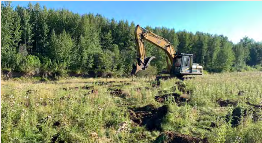
Site Preparation at Swan River First Nation
